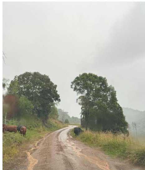
Image 4 Pokolbin Mountains Road water guttering example 2
