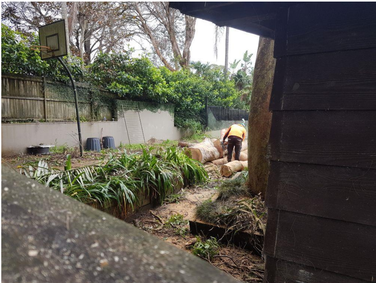
Photo above: Illegal tree removal at 23 Balfour Street, 29 September 2024, taken by W. Palmer.
