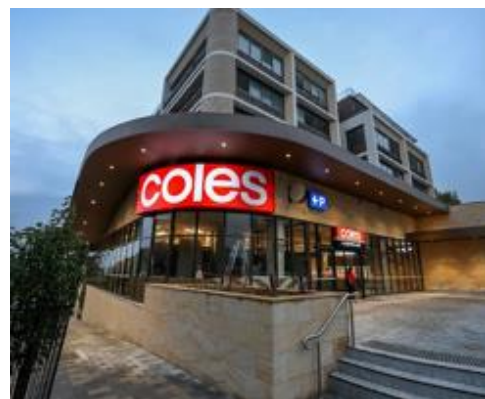
Coles re-development corner of Pacific Highway and Balfour Street
