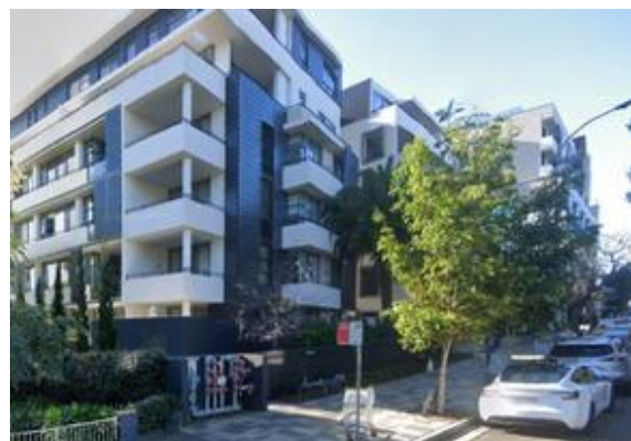
5-6 storey residential flat building in Lindfield Avenue
