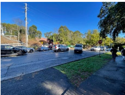
Figure 7. The narrow rail bridge on Havilah Lane, under which is Nelson Road's most direct route to the Pacific Highway, creates a choke point causing delay and friction at the nearby intersection, and further problems at a nearby intersection, resulting in road users experiencing significant delays and some breaking road rules to get around the traffic chaos this creates at peak times. The intersections and the rail bridge are an example of inadequate infrastructure servicing current traffic volumes, which will be exacerbated by the addition of 167 apartments and 251 car spaces proposed in close proximity.
