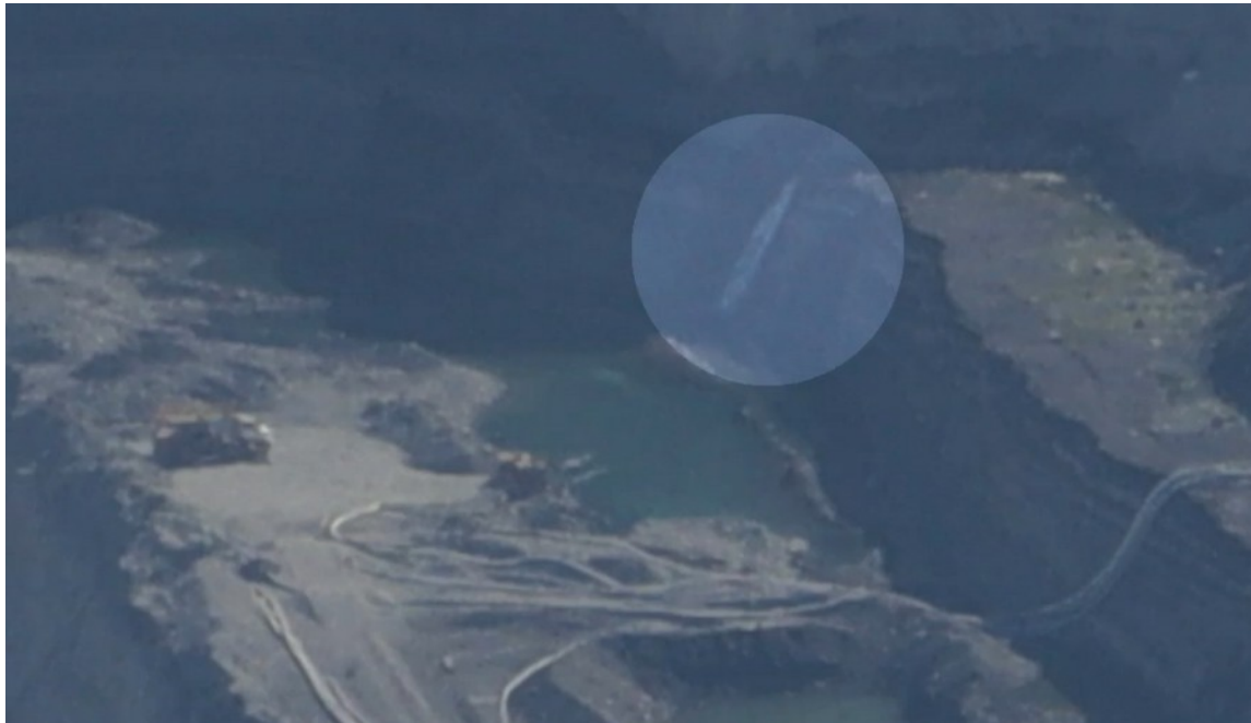
Photo 5: Groundwater waterfall midway up the highwall (MCCC (2024))
