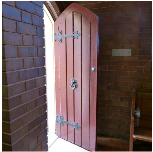
Figures 20 and 21 | Detailing of brickwork, which is darker in tone than bricks in the surrounding walls, around paired windows lighting the aisles (left); boarded door with decorative wrought metal hinges and handle at the rear of the church (right).
