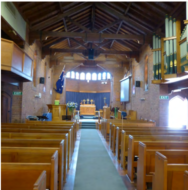
Figures 22 and 23 | Looking east along the nave towards the apse (left); exposed timber roof trusses supported off corbelled wall brackets- timber boards have been installed between the trusses to line the underside of the roof (right). The heads of windows are linked by a string course.
