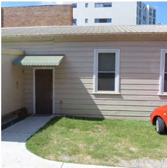
Figures 44 and 45 | Rusticated timber weatherboards and recent windows on the northern side of the Hall (left); skillion roofed northern section of the Hall. The difference in roof level between the original section of the Hall (circa 112 to 1926) and the later eastern addition is clearly apparent, as is the differing condition of roof linings.
