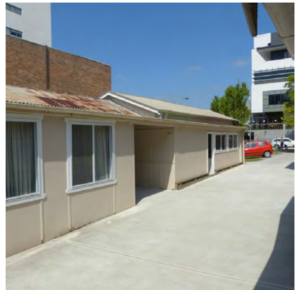
Figures 44 and 45 | Rusticated timber weatherboards and recent windows on the northern side of the Hall (left); skillion roofed northern section of the Hall. The difference in roof level between the original section of the Hall (circa 112 to 1926) and the later eastern addition is clearly apparent, as is the differing condition of roof linings.
