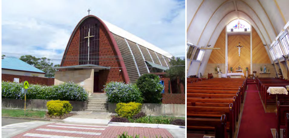
Figures 75 and 76 | St Bernard's Roman Catholic Church at Botany, designed by Kevin Curtin and completed in the first half of the 1950s, demonstrates how architects experimented with advanced structural techniques, in this case tensioned parabolic arches, to determine the form and spatial character of the buildings [Roy Lumby Photographs]
