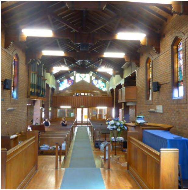
Figures 27 and 28| Looking west along the nave from the chancel. The organ can be seen at left, with the cantilevered timber choir opposite (left); southern side aisle. The external piers are reflected by rhetorical buttressing pieced by arched openings. Timber bolsters carry the beam supporting the wall section, which is lined with acoustic panels, between aisle and nave. The vertical timber boards at right above the pews form part of the low balustrade wall across the gallery at the western end of the church (right)
