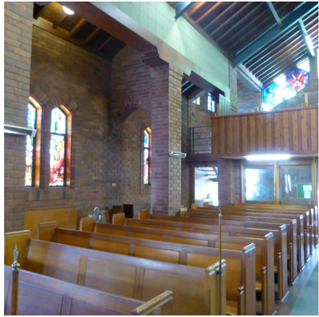
Figures 27 and 28| Looking west along the nave from the chancel. The organ can be seen at left, with the cantilevered timber choir opposite (left); southern side aisle. The external piers are reflected by rhetorical buttressing pieced by arched openings. Timber bolsters carry the beam supporting the wall section, which is lined with acoustic panels, between aisle and nave. The vertical timber boards at right above the pews form part of the low balustrade wall across the gallery at the western end of the church (right)
