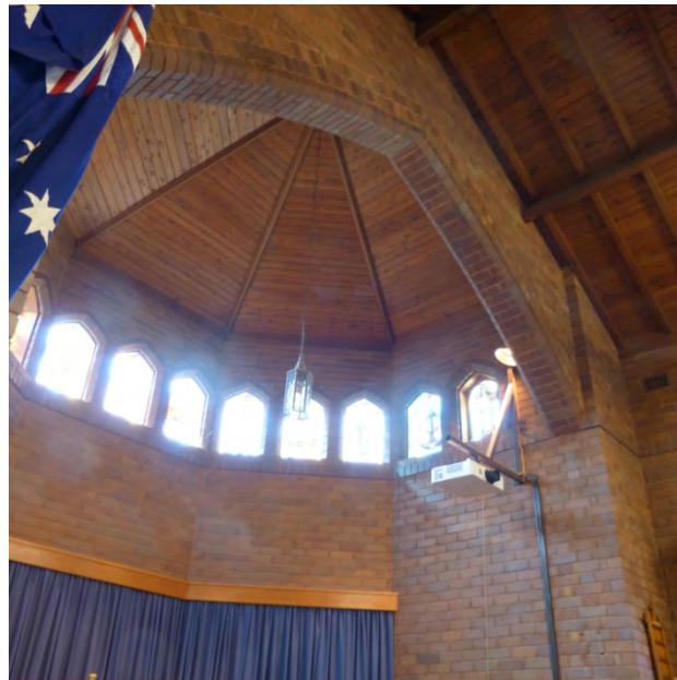
Figure 26 | Timber ceiling lining above the sanctuary. The shallow arch separating the apse from the nave is emphasised by contrasting molded bricks.
