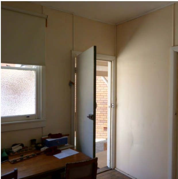
Figures 55 and 56 | Details of the Vestry interior - fibrous plaster wall and ceiling linings with joints covered by slender timber mouldings, polished pine floor boards and an enameled hand basin in one corner.
