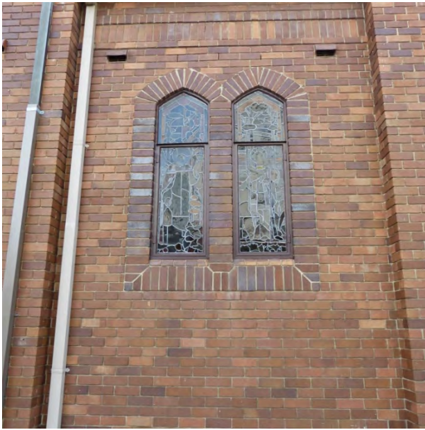
Figures 20 and 21 | Detailing of brickwork, which is darker in tone than bricks in the surrounding walls, around paired windows lighting the aisles (left); boarded door with decorative wrought metal hinges and handle at the rear of the church (right).
