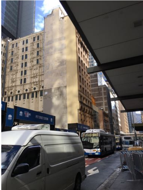
Figure 5: NSW Masonic Club, southern elevation, with Pitt Street North (OSD) hoarding in the foreground. 2018. Note the row of circular highlights with bay windows below indicating the location of the Grand Dining Room.
