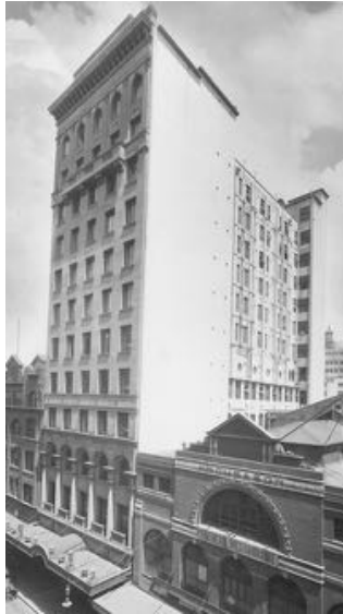
NSW Masonic Club, Castlereagh Street Elevation. Circa 1930. Photo NSW Masonic Club archives.
