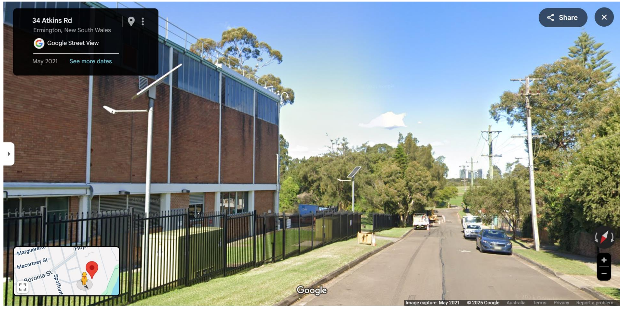
Google Maps Street View. Padmount substations no.s 25495 & 28866.
