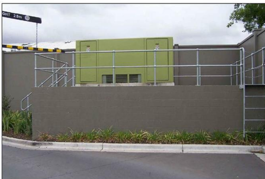
Figure 51 - Example substation raised above 1:100 flood level
