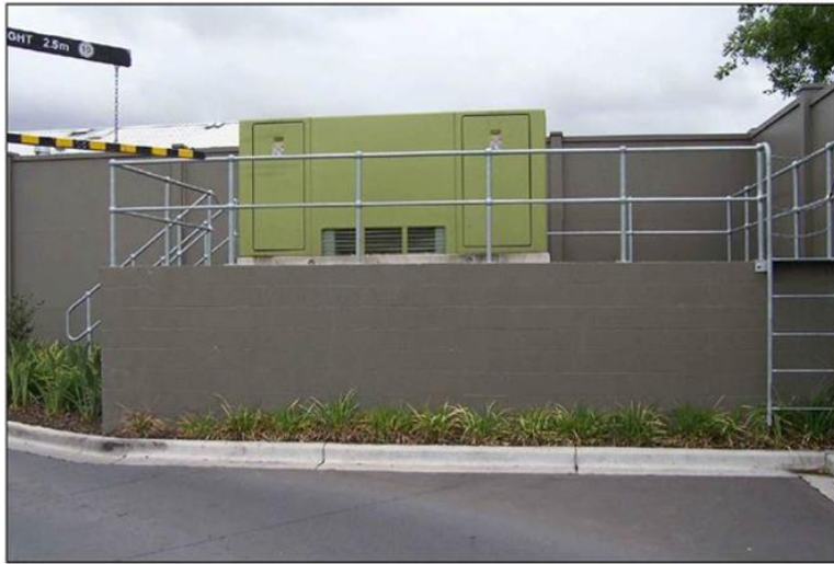
Figure 51 - Example substation raised above 1:100 flood level
