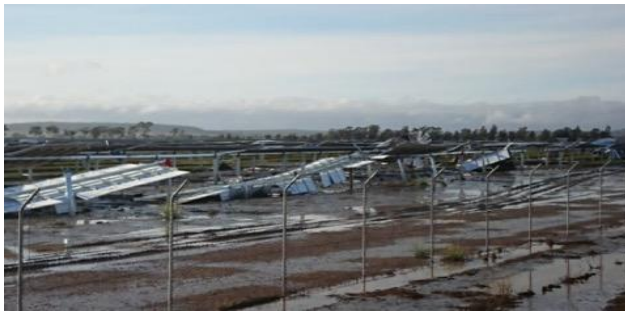
Storm damage to a PV solar works
