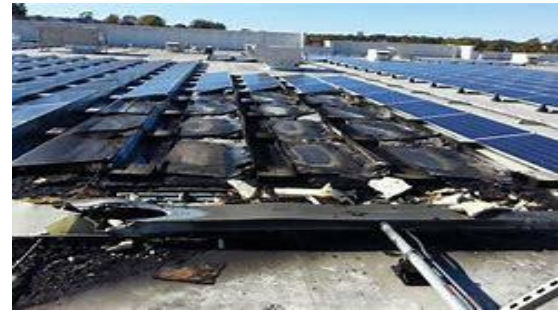
Fire damage to a PV solar works
