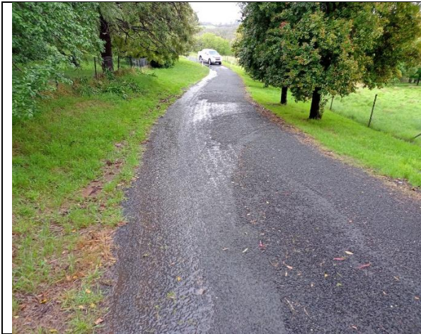
Photo x .4: Road bitumen wash 2
