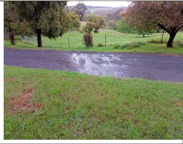
Photo x .5: Road bitumen wash 3
