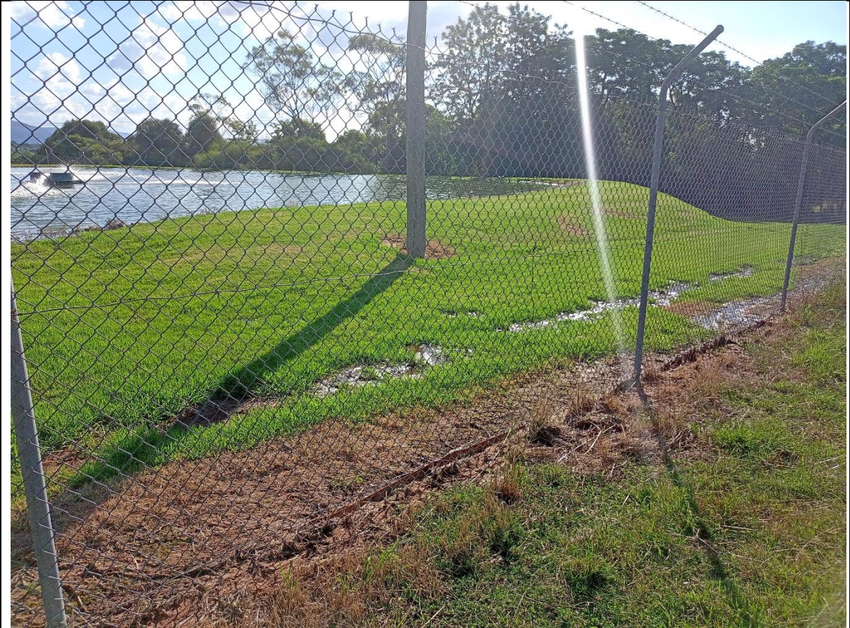
Photo x .1: Sewerage Treatment Pond overflowed
