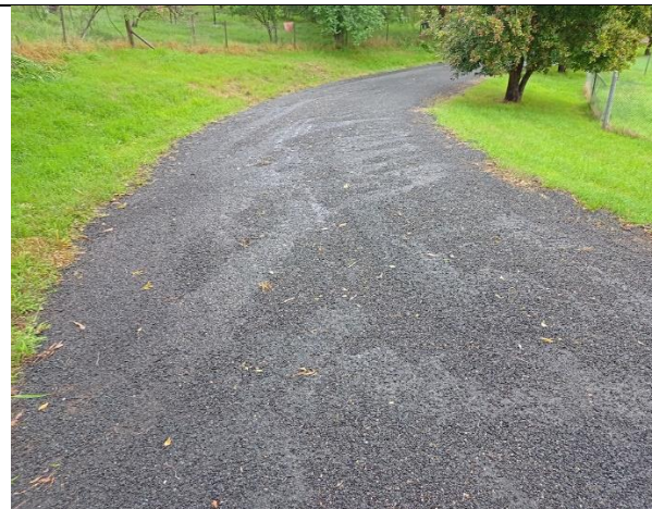
Photo x .3: Road bitumen wash 1
