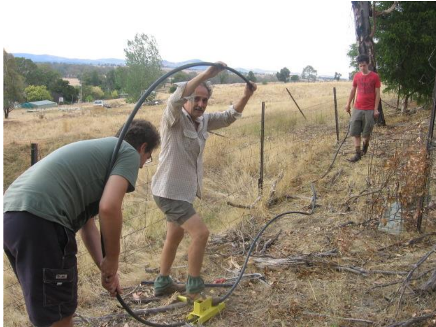
Stuart, John and Andrew splitting poly pipe to go over barbed wire strands.
