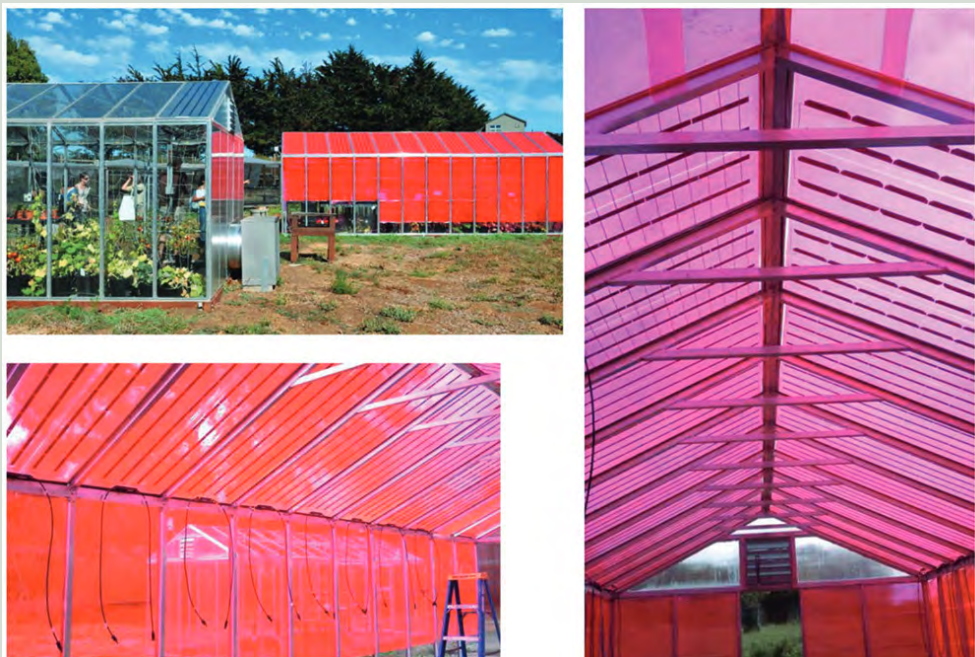
Figure 3: Luminescent Solar Concentrator (LSC) PV integration for greenhouse
