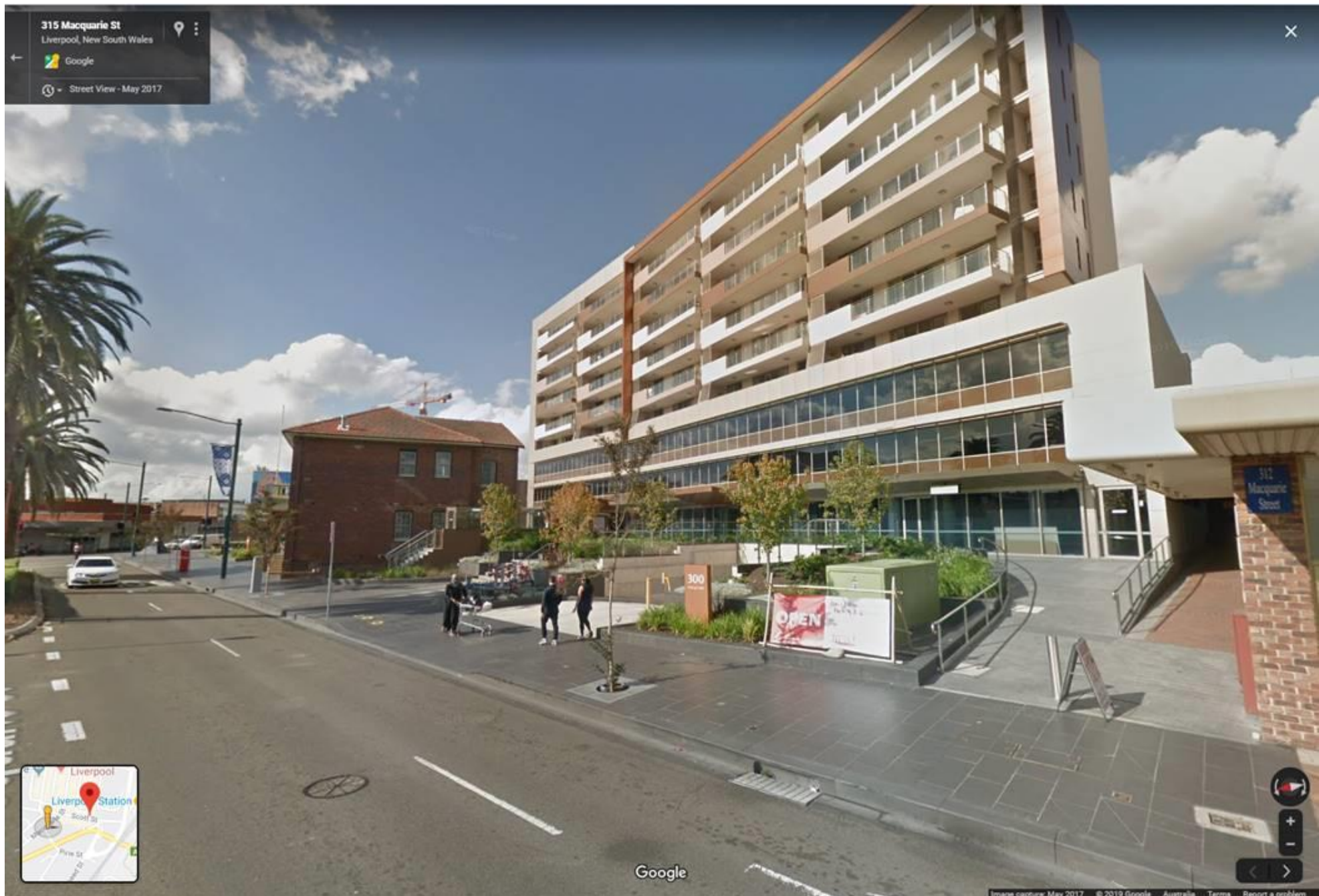
Padmount substation no. 33223 located on Lot 201 DP 1224084 with frontage to Macquarie Street
