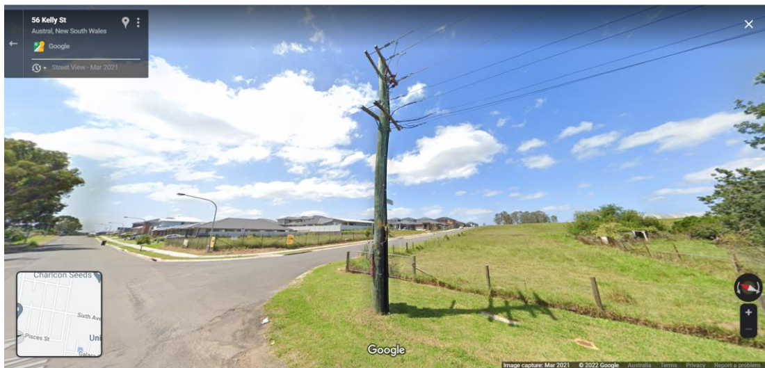
Overhead power lines are progressively undergrounded as subdivisions progress. Source: Google Maps Street View.
