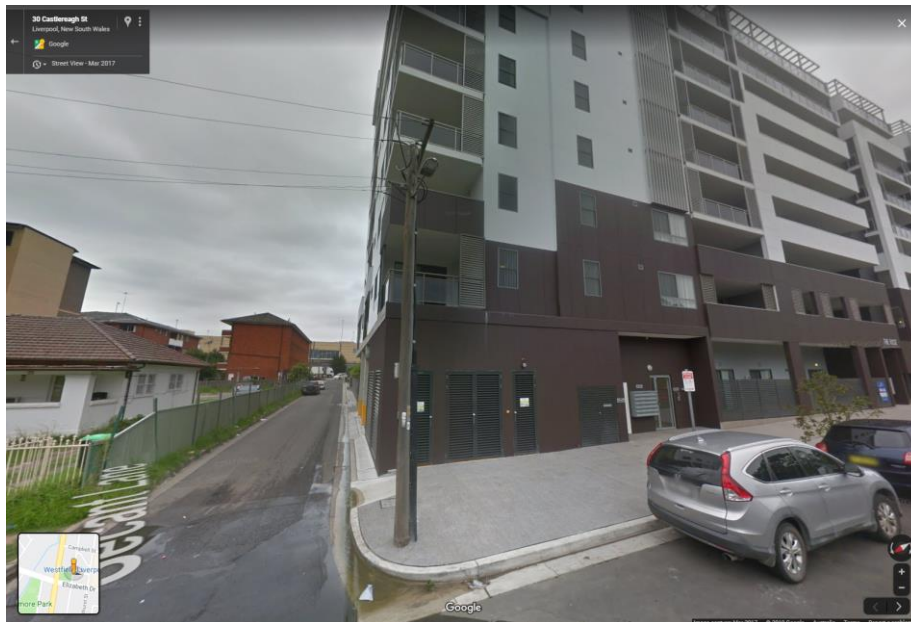
Indoor substation at 32 Castlereagh Street Liverpool. Source: Google Maps Street View.
