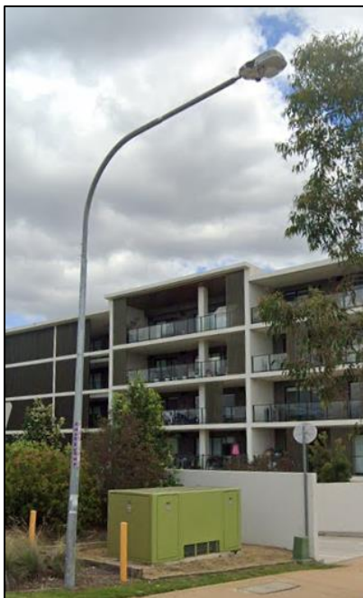
Low voltage pillar, streetlight column and padmount substation at Goodison Street North Kellyville. Source: Google Maps Street View.
