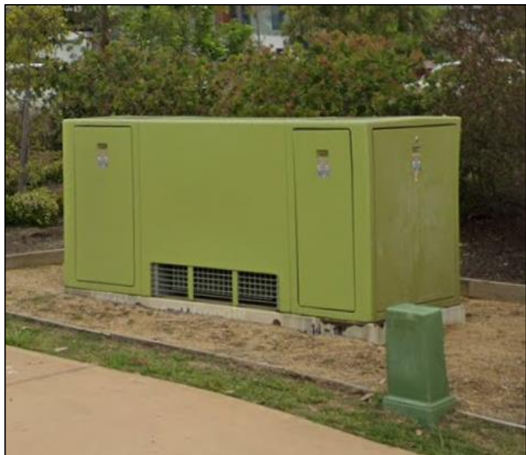
Low voltage pillar, streetlight column and padmount substation at Goodison Street North Kellyville. Source: Google Maps Street View.
