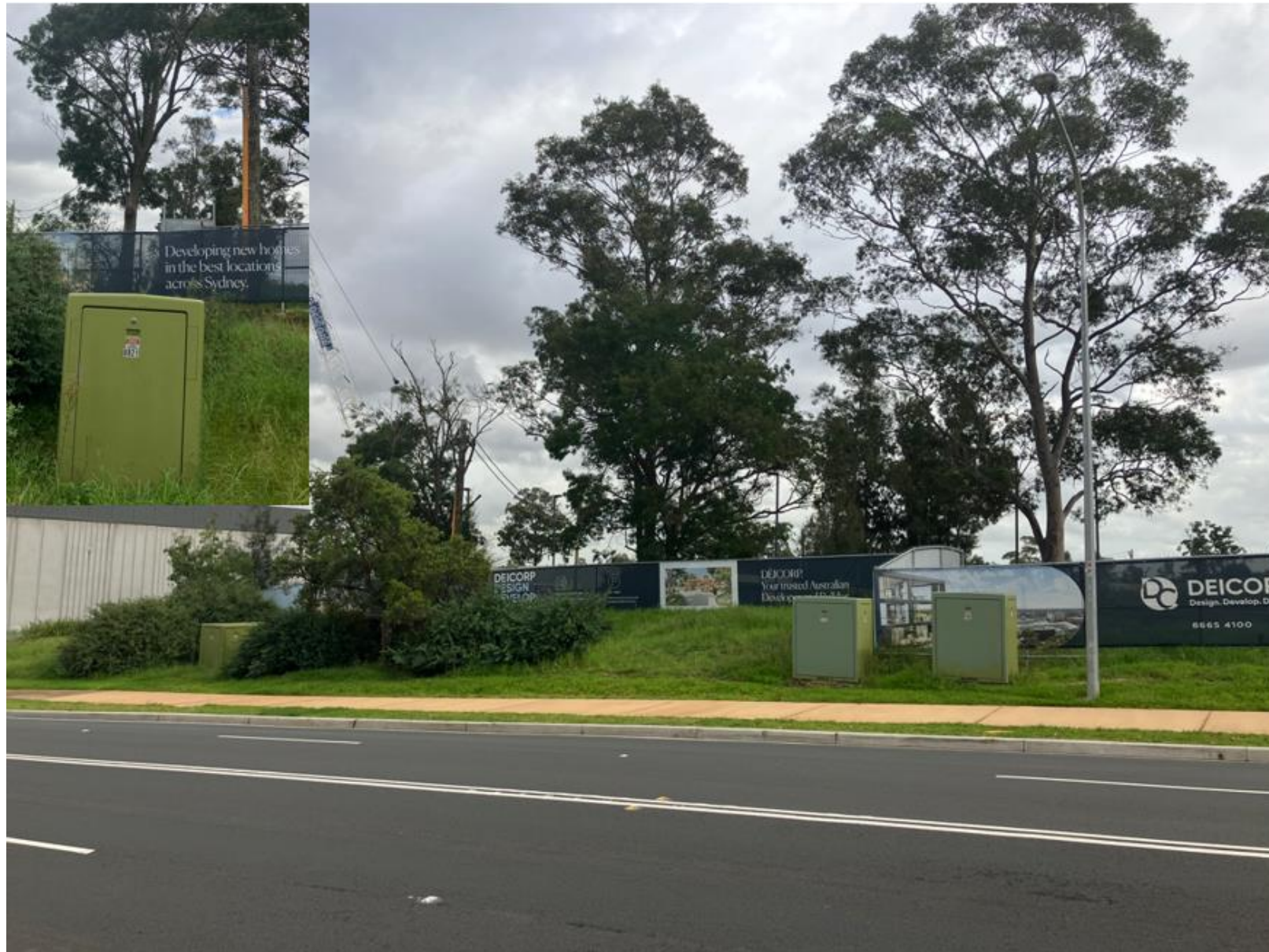
Photograph 15/03/2024. From padmount substation no. 8821 there appears to be extended low voltage overhead service conductor for temporary builder's supply traversing the site which is not shown in the Site Plan from Endeavour Energy's G/Net Master Facility Model.
