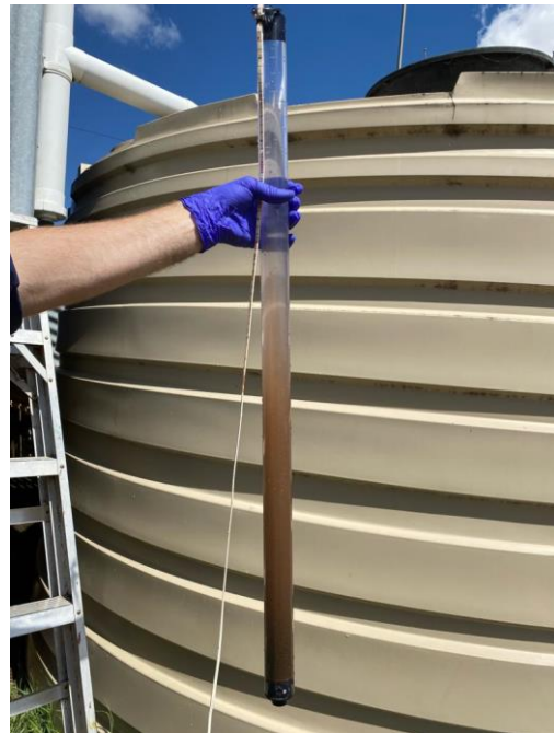
Tank cleaned 10 months prior to this photo being taken, it was also cleaned twice in the previous 24mths.
