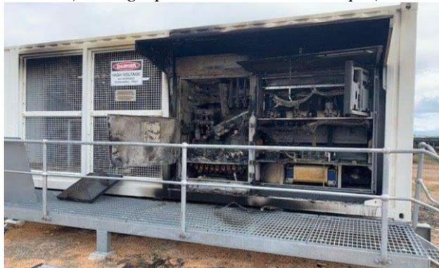
*(Photograph 2: Fire damaged Inverter post fire event)*
