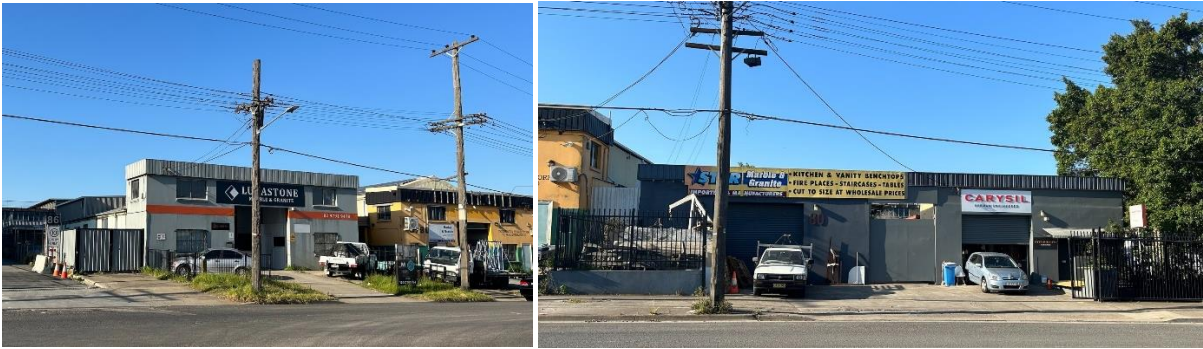
Figure 3: Photos of the existing buildings at 84, 82 & 80 Gow Street, Padstow (left to right)
