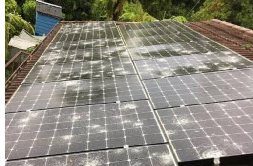
Solar panels damaged by hail
