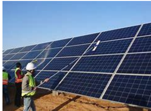
Cleaning PV solar panels
