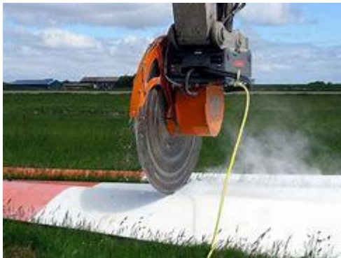
Cutting up end-of-life wind turbine blades
