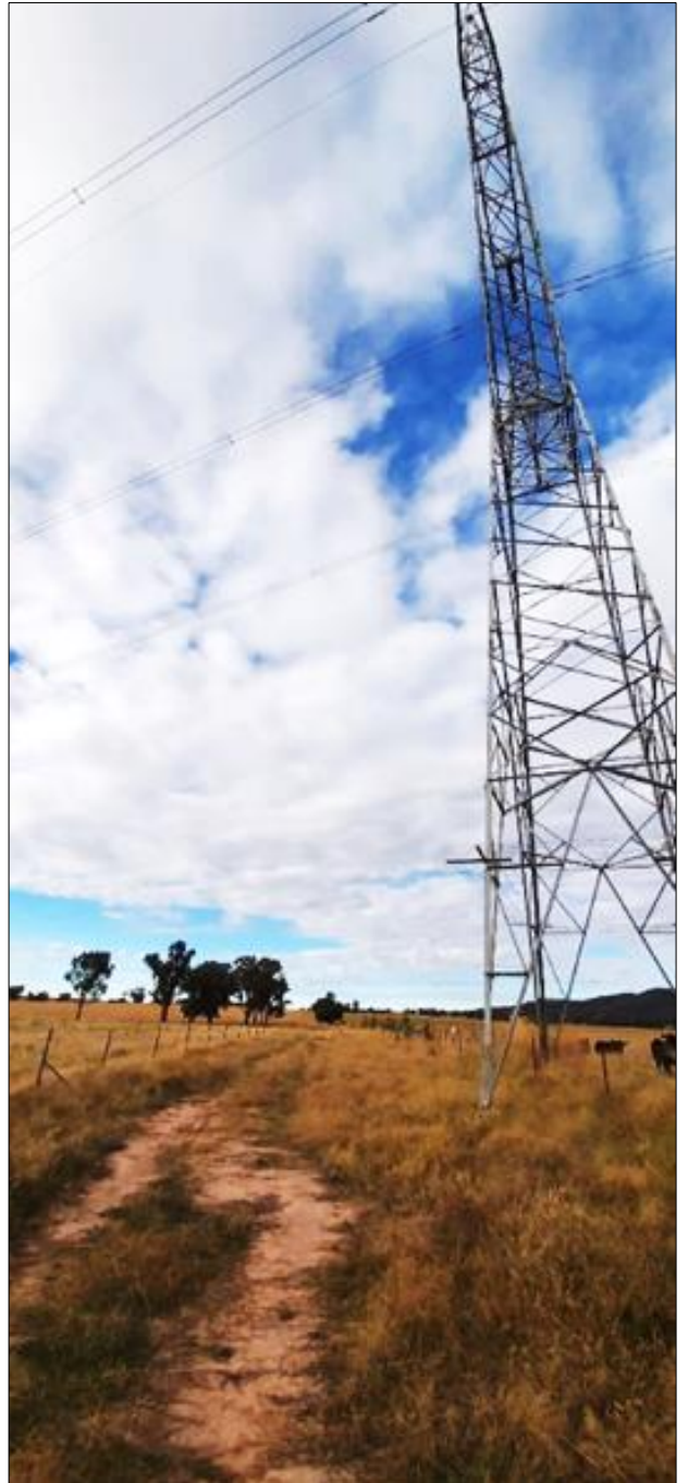
Photo 2. SWANS placement of tower hindering laneway & machinery access
