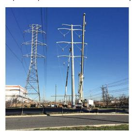
"As the roughly 90-ft-tall [33m] lattice structures are taken down, they are replaced with monopole structures that will carry the new 345-kV lines. PSE&G is using monopoles because they are quick to install, have a small footprint and are less expensive, Tkachuk says.
