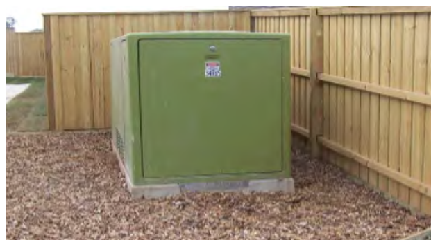
Correctly maintained padmount surrounding area
