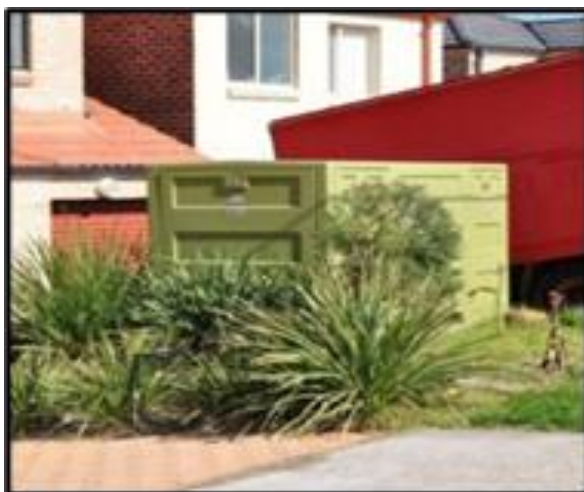
Padmount substation
