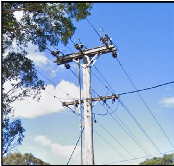
High and low voltage overhead mains
