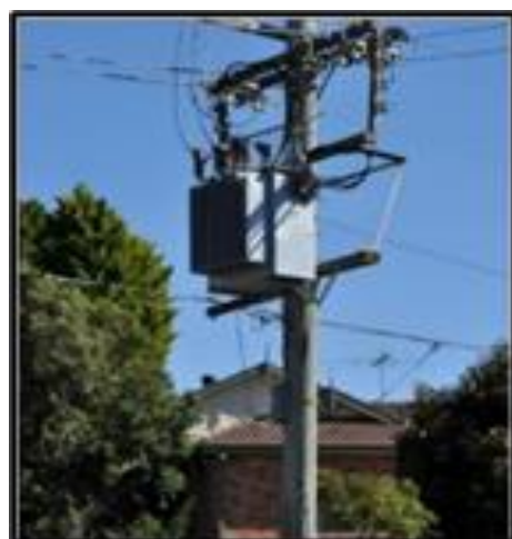
Pole mounted substation
