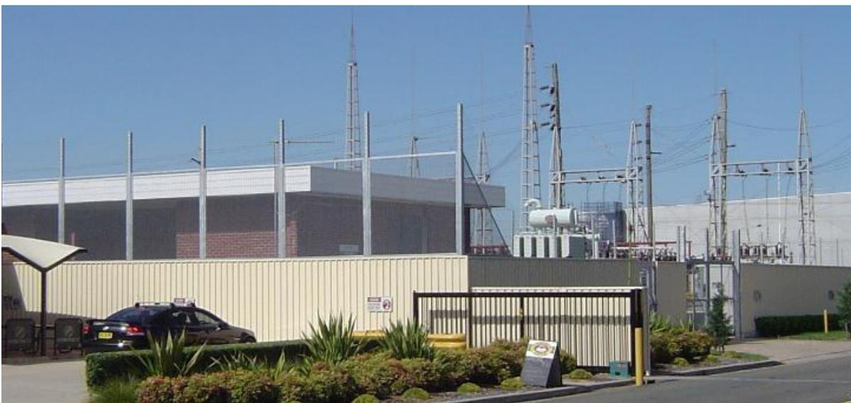
Endeavour Energy's Seven Hills Zone Substation is an 'outdoor' design. Note height of fencing due to adjacent 'climb point' created by the seating and awning.
