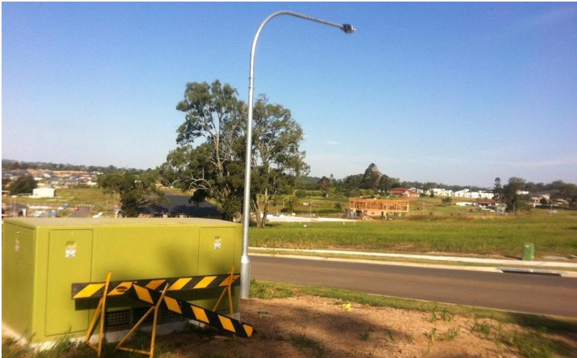
Padmount substations are converters of electricity, reducing the high voltages for street lighting and to the end user whilst low voltage pillar boxes are distribution junction points. These structures also mean underground cables are nearby. Digging activities and planting of trees or shrubs should not occur near them.
