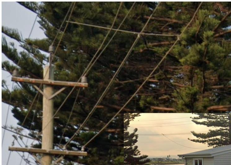
The mid span / suspended low voltage overhead service conductor for an existing dwelling avoids the nearby trees. The new development of the site will likely need to utilise an extended low voltage overhead service conductor coming from the pole on the road verge to a customer owned / private pole located within 1 metre of the front boundary. Source: Google Maps Street View.
