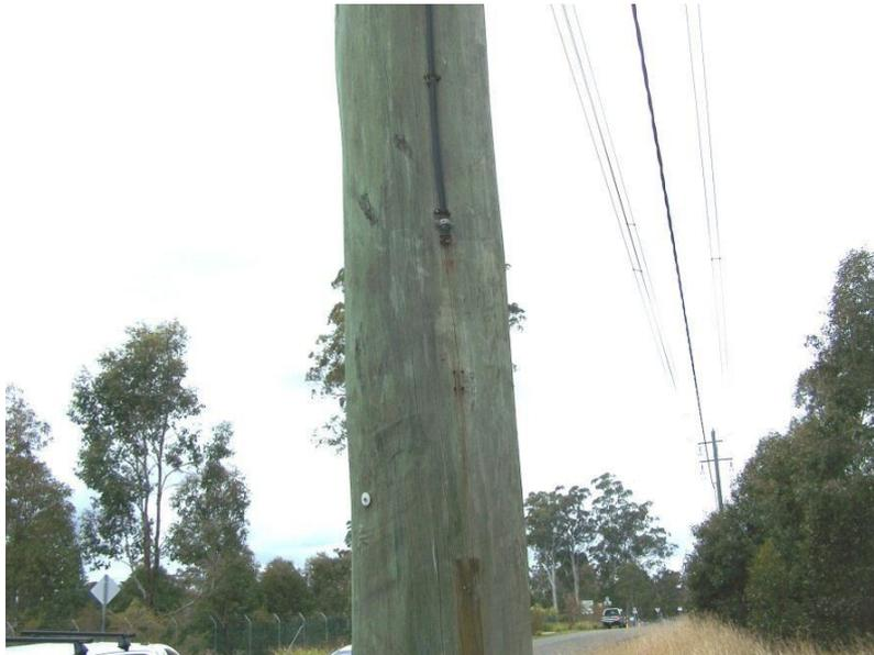
Copper thieves cutting and taking earths from power poles means there is inadequate connection to the earth placing persons and the electricity network at risk. This example occurred in Prospect NSW part of Endeavour Energy's franchise / network area. Crime Stoppers is urging anyone with information about copper theft in their area to report it anonymously to Crime Stoppers on 1800 333 000.
