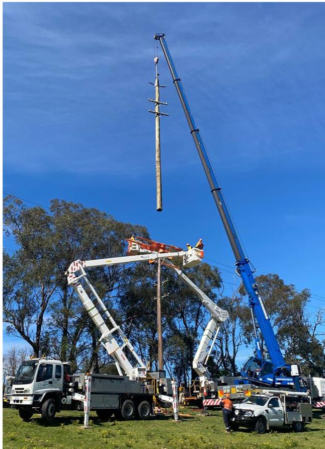
The equipment required for pole replacements can include up to a 60 ton crane, franna crane, large elevating work platform and lifter borer.
