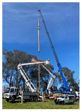
The equipment required for pole replacements can include up to a 60 ton crane, franna crane, large elevating work platform and lifter
