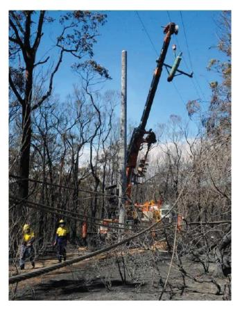
Endeavour Energy crews replacing a burnt timber pole with a concrete pole after the September 2013 bush fire at Winmalee NSW.
