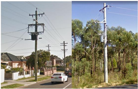
Pole mounted substation no. 914 in Blaxcell Street, Guildford NSW has 79 customer connection points servicing 119 premises in an urban context which is at the upper end of the number of premises able to be serviced. In contrast pole mounted substation no. 26132 in Baaners Lane Little Hartley NSW in a non-urban context only services a single rural property. Source: Google Maps Street View.
