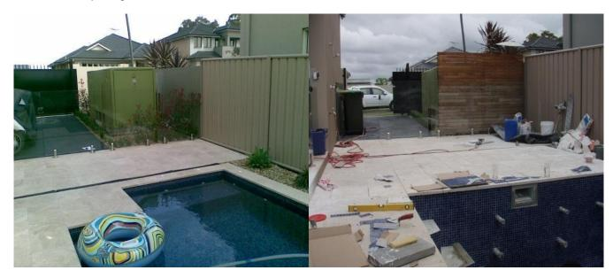
Before and After. This swimming pool in Endeavour Energy's network area at Middleton Grange NSW had to be modified to comply with the restriction for the padmount substation on the use of land in relation to swimming pools.
