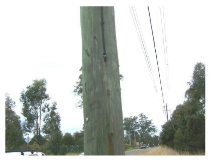
Copper thieves cutting and taking earths from power poles means there is inadequate connection to the earth placing persons and the electricity network at risk. This example occurred in Prospect NSW part of Endeavour Energy's franchise / network area. Crime Stoppers is urging anyone with information about copper theft in their area to report it anonymously to Crime Stoppers on 1800 333 000.
