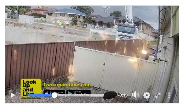
In December 2022 a concrete boom truck in Western Sydney came into contact with a 33,000 volt / 33 kilovolt high voltage overhead powerlines causing an electrical explosion that energised the immediate area with potentially fatal consequences. Thankfully no one was killed or seriously hurt. Source: Too often Endeavour Energy (NSW) is... - Endeavour Energy | Facebook
