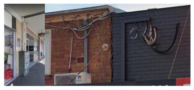
Example of 'awning' overhead power lines coming from a low voltage pillar on the road verge rising to through a duct and then through or above the awnings to the customer connection points for the premises. Source: Google Maps Street View.
