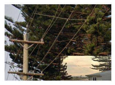
The mid span / suspended low voltage overhead service conductor for an existing dwelling avoids the nearby trees. The new development of the site will likely need to utilise an extended low voltage overhead service conductor coming from the pole on the road verge to a customer owned / private pole located within 1 metre of the front boundary. Source: Google Maps Street View.
