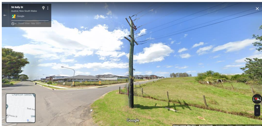
Overhead power lines are progressively undergrounded as subdivisions progress. Source: Google Maps Street View.
