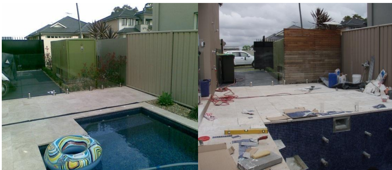
Before and After. This swimming pool in Endeavour Energy's network area at Middleton Grange NSW had to be modified to comply with the restriction for the padmount substation on the use of land in relation to swimming pools.
