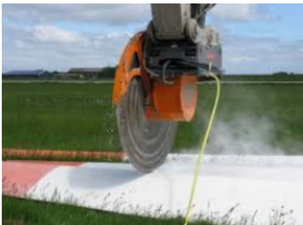
Figure 4 Decommissioning, and the shedding of residue Bisphenonyl A into the environment, from page 32 of Appendix S, Decommissioning and Rehabilitation
