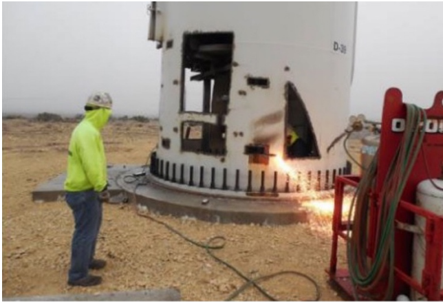
Figure 24 | Oxy-acetylene cutting preparation of tower base
