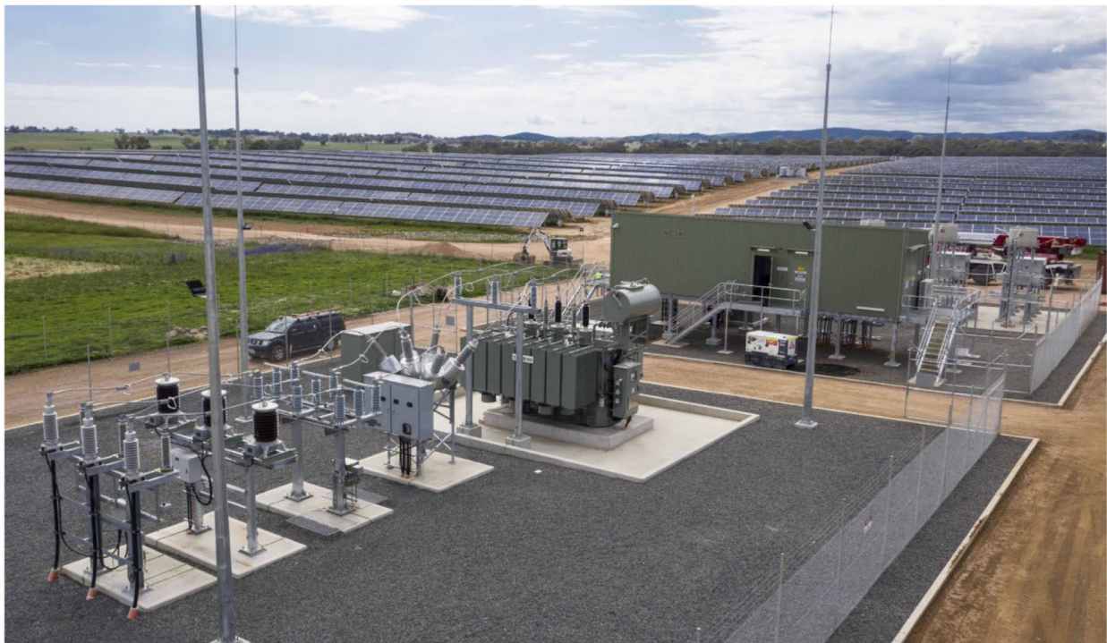
Figure 3-5 Typical substation; Molong Solar Farm (33/66kv connection).
