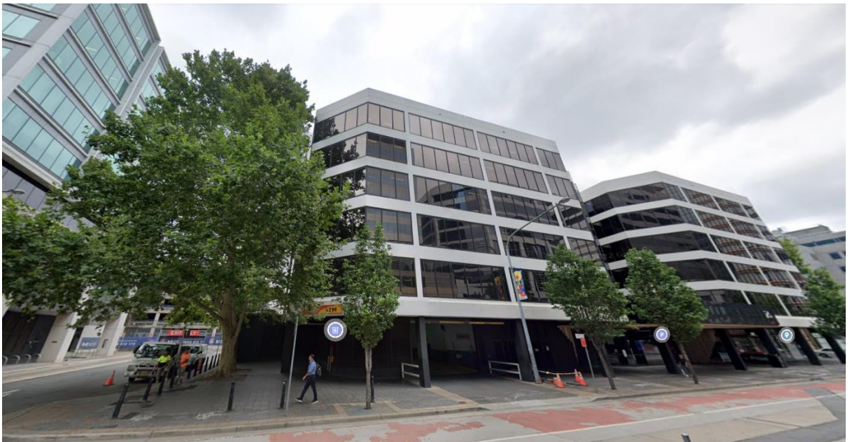
Figure 3 75 George Street, looking east from Smith Street (Macquarie Lane shown left, existing vehicular access shown in middle from Smith Street)
