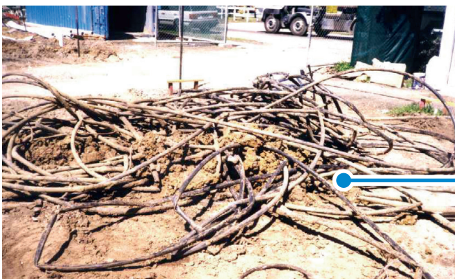
Sub-ducts and cables laying on the construction site, pulled out by an auger.
