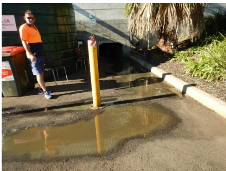
5. Discoloured, odorous leachate flowing through stormwater pipe under building
