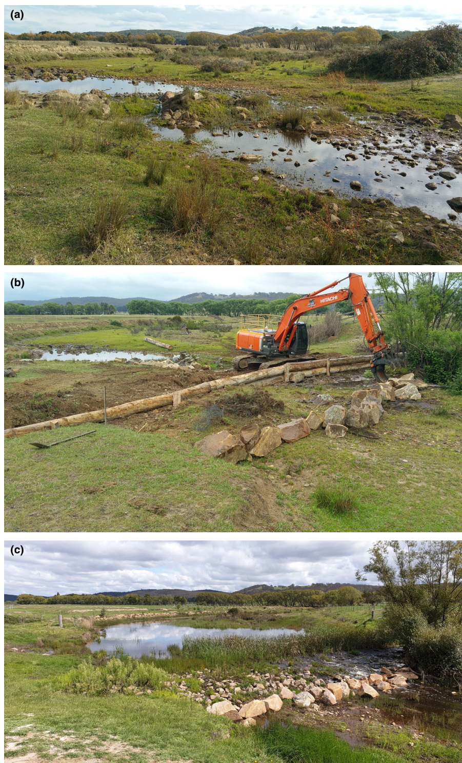
Figure 5. A typical Mulloon Rehydration Initiative site (WVM1): (a) pre-works; summer 2018; (b) site works summer of 2018; (c) initial recovery – autumn 2020. The hydrological and ecological outcomes of these constructions are the focus of on-going monitoring. Preliminary results to be published in the near future (Photos by Peter Hazell).
