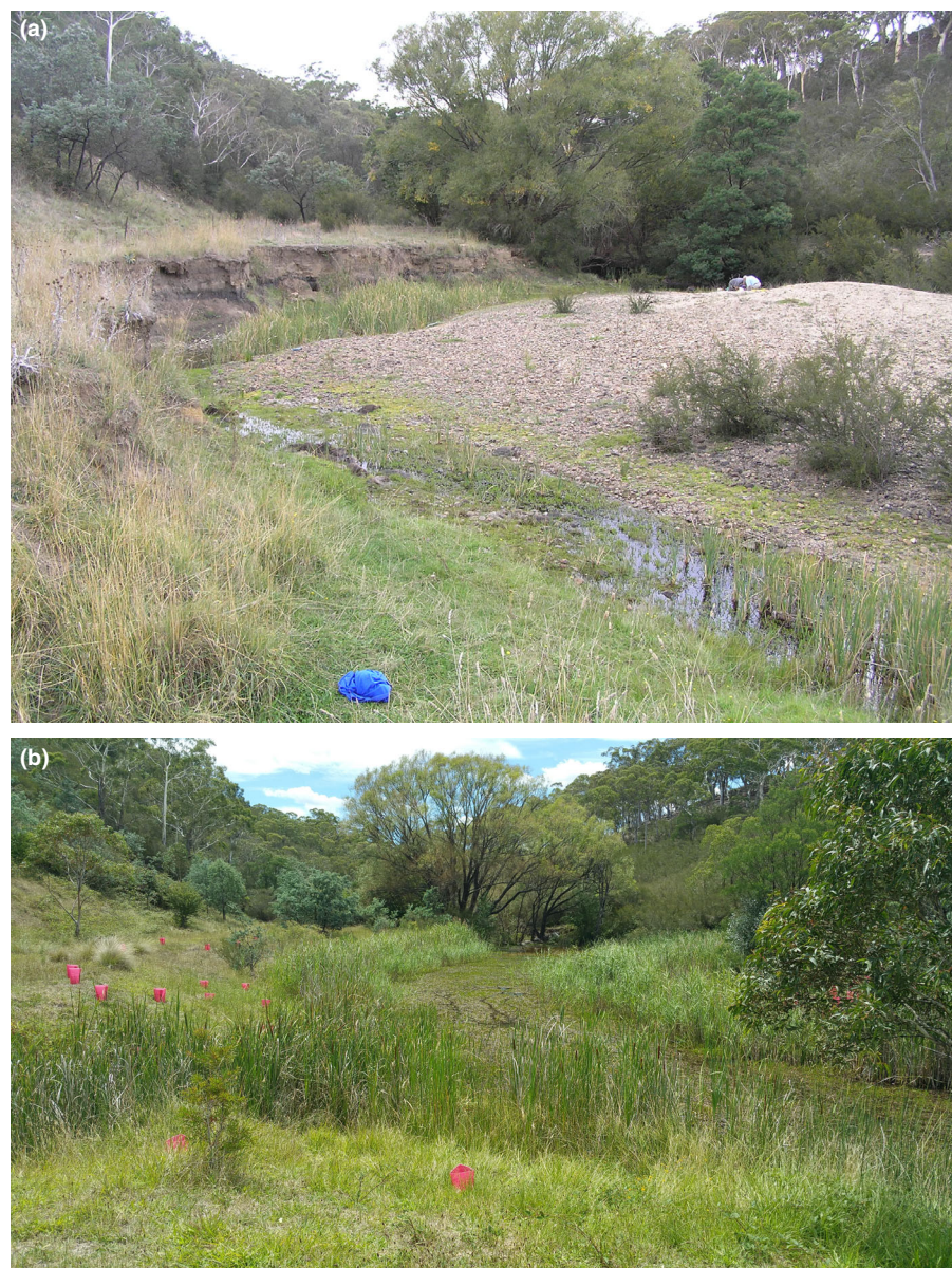
Figure 4. (a) A typical degraded pilot site showing the incised stream bank and lack of ponding (March 2006). (b) The same reach ("Peter's Pond") by February 2018 showing extensive stream bank revegetation and extensive ponding following the establishment of a stone-based 'leaky weir'. (Photos by Peter Hazell).
