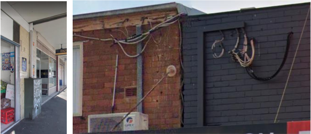
Example of 'awning' overhead power lines coming from a low voltage pillar on the road verge rising to through a duct and then through or above the awnings to the customer connection points for the premises. Source: Google Maps Street View.
