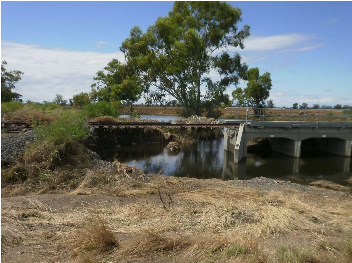
Culvert north of P1 “A more recent upgrade and current design”
