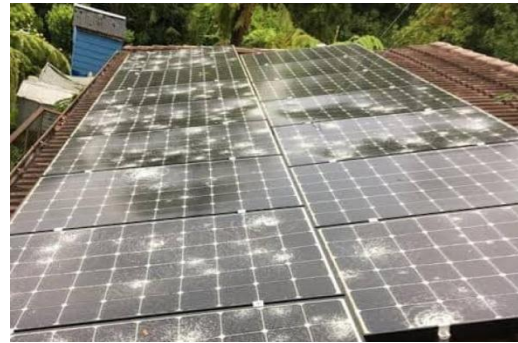
Solar panels damaged by hail
