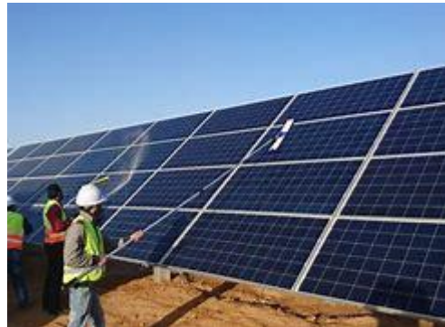
Cleaning PV solar panels
