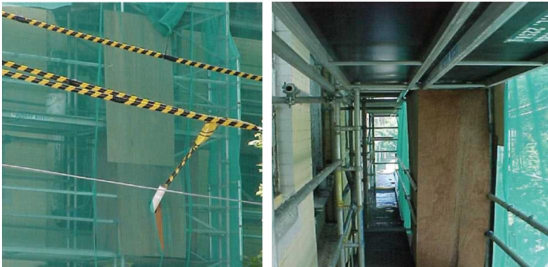
**Figure 11 – Enclosure of overhead powerlines**
