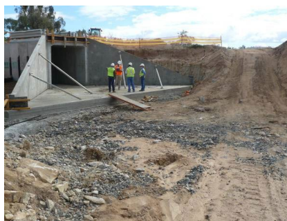
New boxed culvert tunnel under construction
