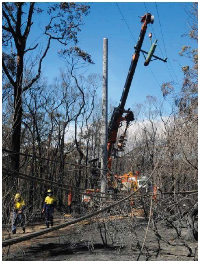
Endeavour Energy crews replacing a burnt timber pole with a concrete pole after the September 2013 bush fire at Winmalee NSW. Source: Everyday Endeavours, Staff Newspaper November 2013
