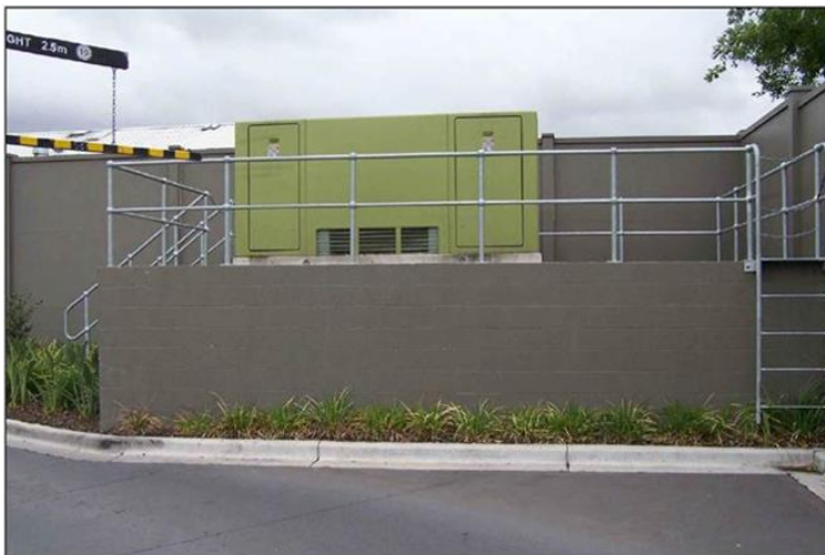
Figure 51 - Example substation raised above 1:100 flood level
