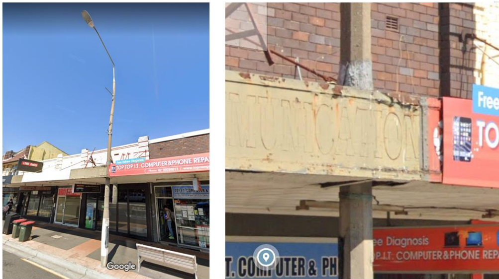
The street awning is inappropriately constructed around the streetlight column. Source: Google Maps Street View.
