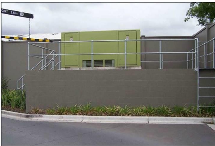
Figure 51 - Example substation raised above 1:100 flood level
