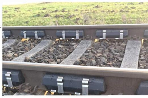
also no need to dismantle the elements when tamping or grinding the tracks. Control and/or survey work of rail fastenings are not affected or hampered.
