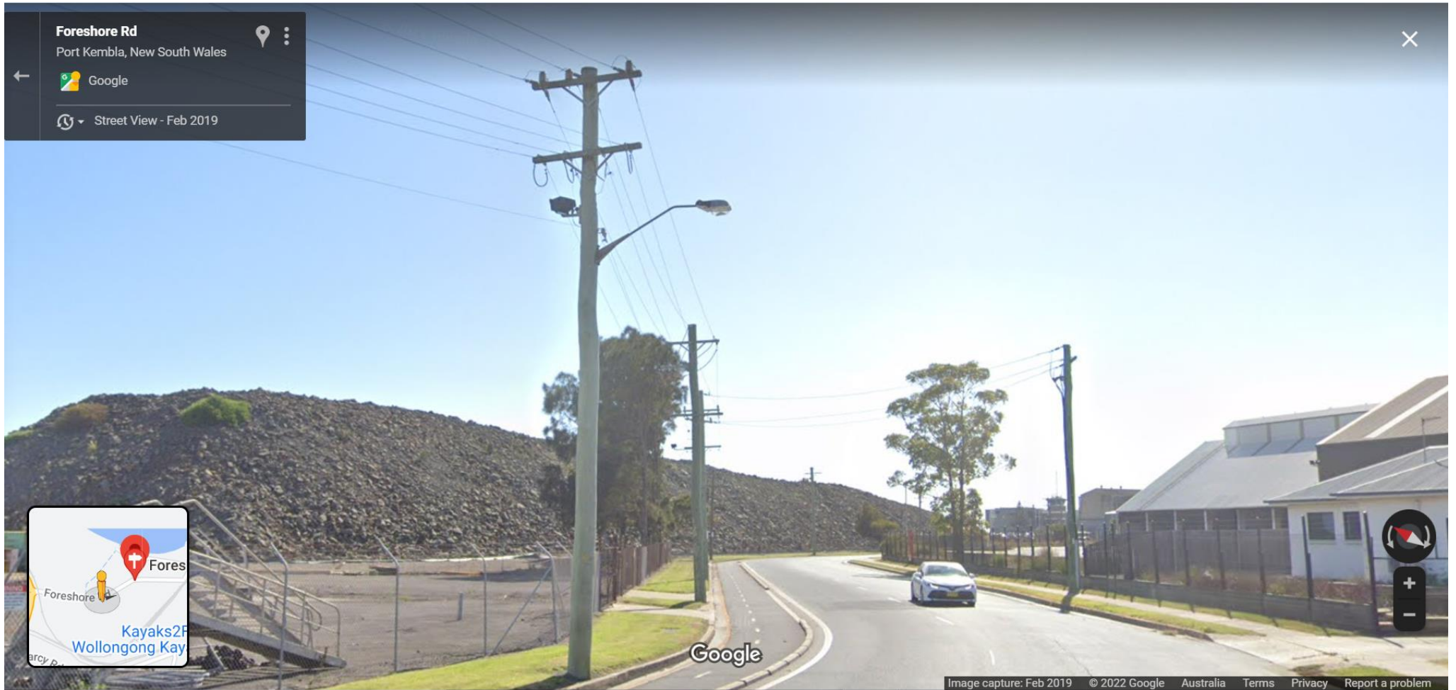
Google Maps Street View. Low voltage and 11,000 volt / 11 kilovolt (kV) high voltage overhead power lines to the Foreshore Road frontage.
