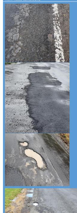
There are poor road conditions on all corridors, including potholes and very poorly constructed temporary hot and cold mix patches across a large percentage of the corridor. These features create hazards for motorists and increase the risk of traffic incidents, vehicle wear and tear and present significant challenges relating to interface risks with pedestrians and motorists.
