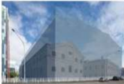
V02: Pier Street northern boulevards looking SW
