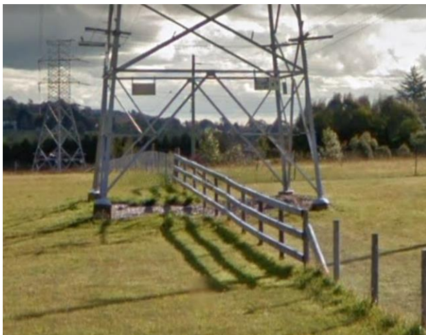
Examples of poor subdivision of easements restricting access and working area around the structures Source: Google Maps Street View.
