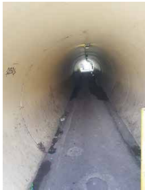
Existing underpass - Internal.
