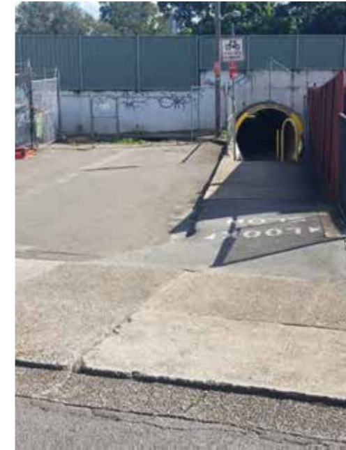
Existing approach on eastern side.
