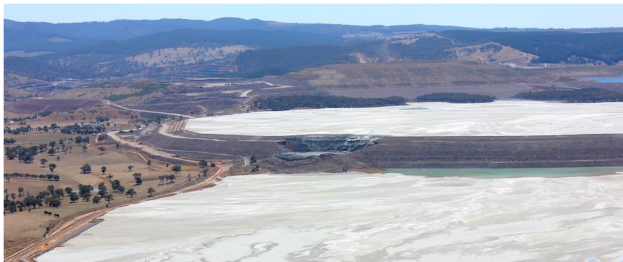
Tailings Dam Failure, March 2018, Cadia, NSW (Source: Riskope, 2018)
