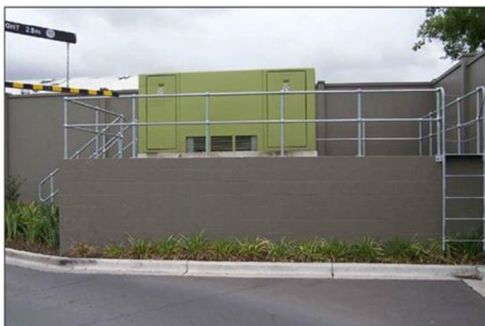
Figure 51 - Example substation raised above 1:100 flood level
